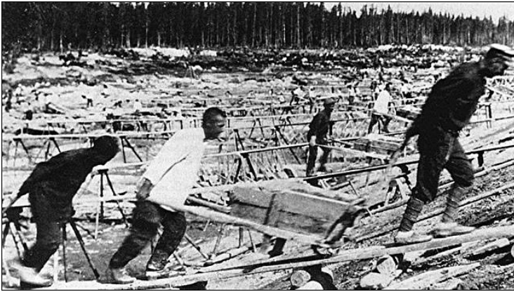
Summer construction on the Moscow-Volga Canal
