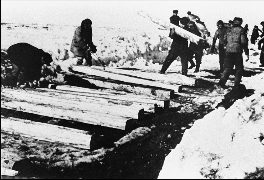
Railroad winter work: Prisoners laying wooden “sleepers”. (Contemporary uncoprighted photo)
